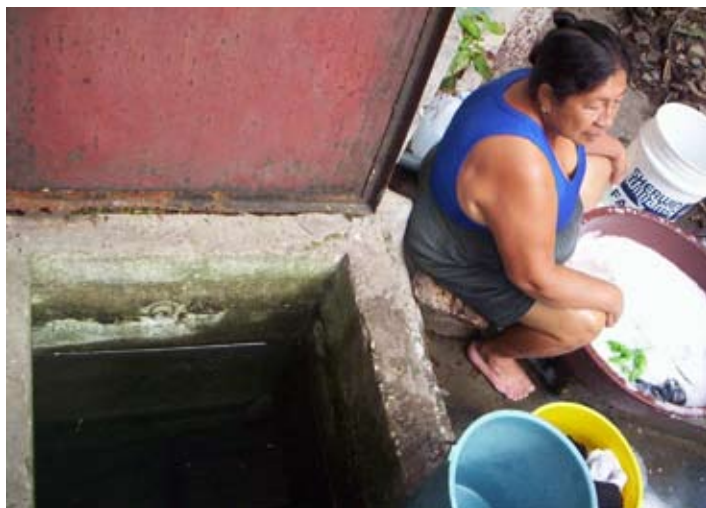
Cistern in Suburbio used for water storage due to unreliable water service. Photo courtesy Observatorio Ciudadano de Servicios Públicos.
