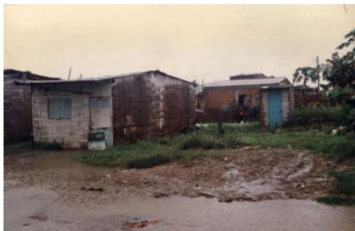
Floods in Guasmo due to the lack of rainwater drainage. Photo courtesy Observatorio Ciudadano de Servicios Públicos.
