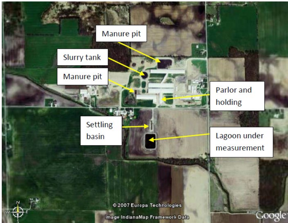
Figure 1-6: Aerial view of IN5A Source: Grant and Boehm (2010a)
